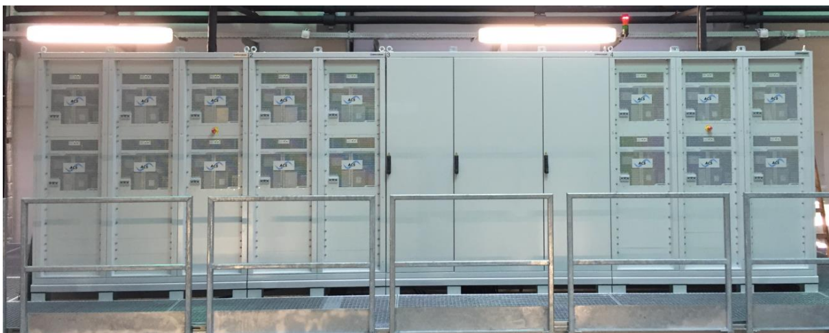
Picture 4: Big scale 800kVA Grid Simulator system for an international Test Facility in Europe
