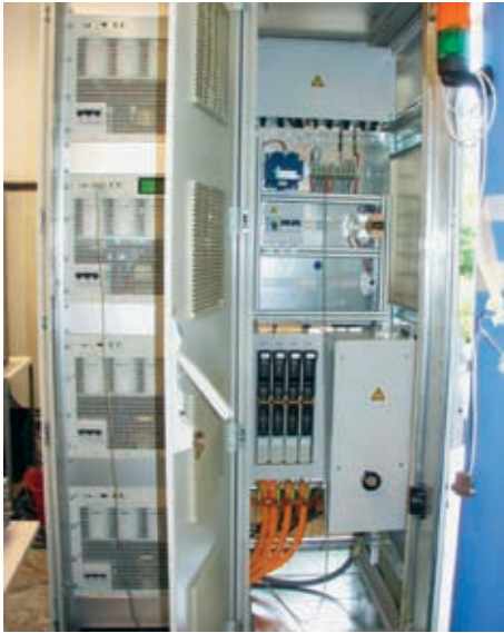
Multiple 32 kW TopCon power supply units in parallel mode, liquid cooled, current range from 0...2000 A
